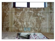
Now you need to work out where to start. Best to find the centre of the wall, use a tile or measuring rod and mark the wall from the centre to the corner and see if the cuts are acceptable. If not make the centre line the centre of tile and see if this gives you a better cut. On this job we worked from the left hand side of window (allowing for out of true reveal). If using mosaics as a border, please read Tip 7.
