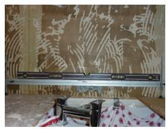
You can now apply adhesive onto the wall using a notched trowel. Do not apply more than  $1m^2$  of adhesive at a time.
