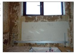
Place tile on the T.M. and start from your line. Tap gently to ensure good contact with the wall and ensuring even gap off the wall, unless you need to level out. Continue tiling along the wall making sure that tiles are level with each other to form a flat surface and using spacers. When first row is completed, you can pencil time of day on the tile, so that after an hour or so you can remove the Tile Master and start on another wall. To tile past end of bath fit leg extensions. Tip 9.
