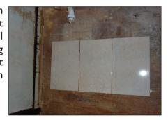
Come down by full tiles before reaching the top of the bath and mark a line on all walls to be tiled. This second line is the first row of full tiles above the bath. This is your datum line which is for guidance only.
