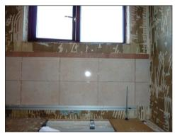
Now, place the T.M. on the bath and adjust legs, so that top edge is level with your datum line. You must check with a spirit level, the line is only for guidance. Place a couple of dabs of tile adhesive on the back of the T.M. to stabilize while adjusting and fixing 1st row of tiles.
